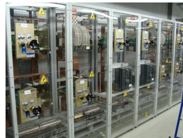
Isolator/contactor/switch gear
